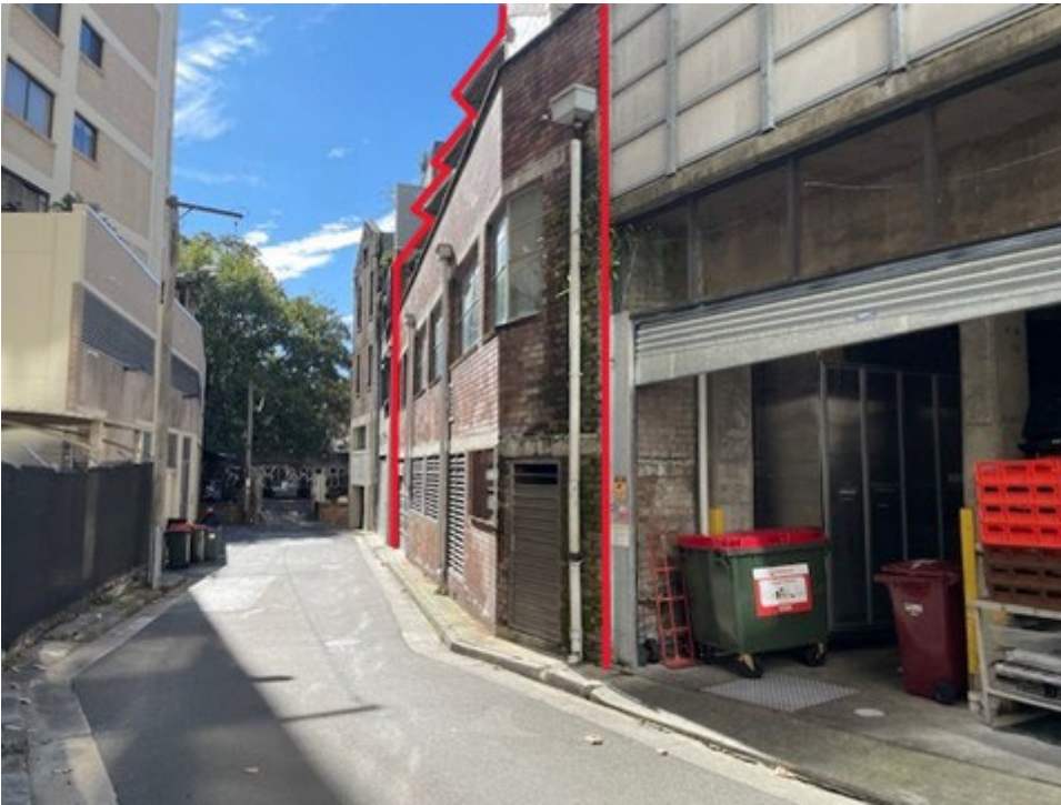
Figure 8. 47 – 51 Riley Street, viewed from the south-west, outlined in red (Busby Lane frontage)
