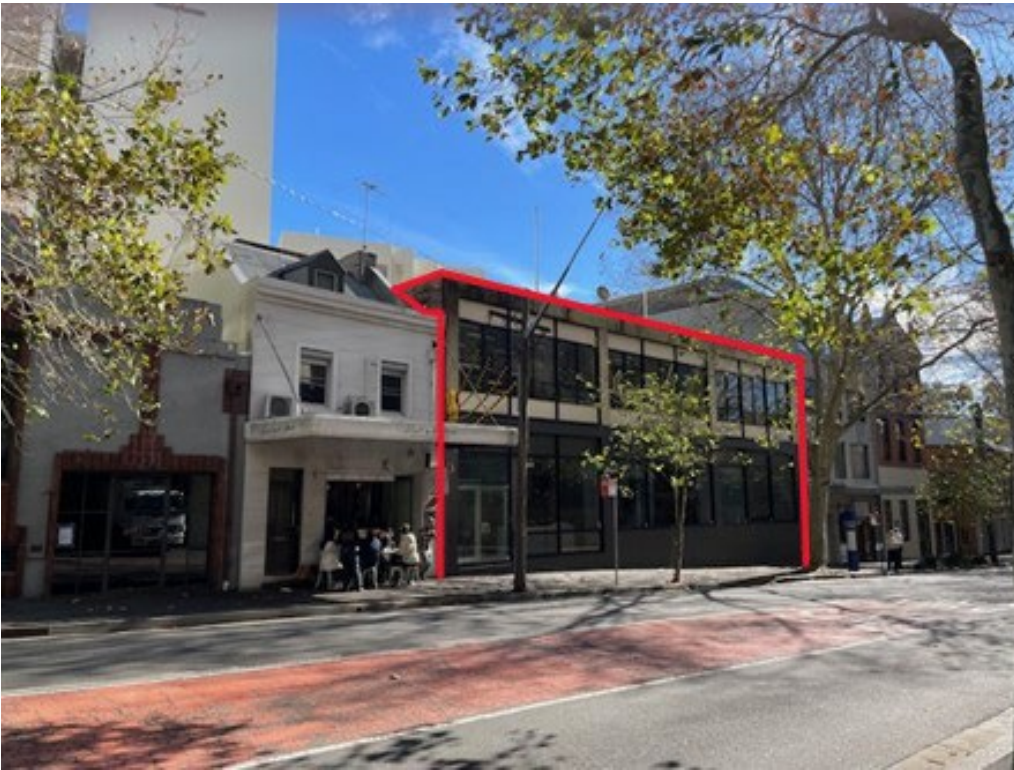
Figure 4. 47 – 51 Riley Street (outlined in red) and adjoining properties, viewed from the south-east (Riley Street frontage)
